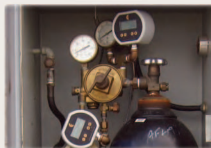
Substation Transformer Nitrogen Blanketing
