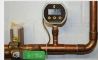
Air Dryer Outlet Temperature
